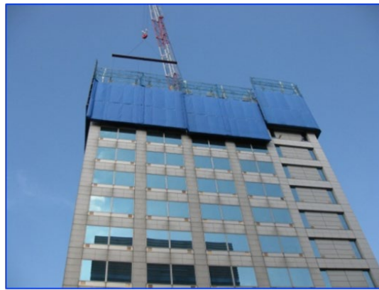
Periphery slide scaffold 1 unit and reshuffle
