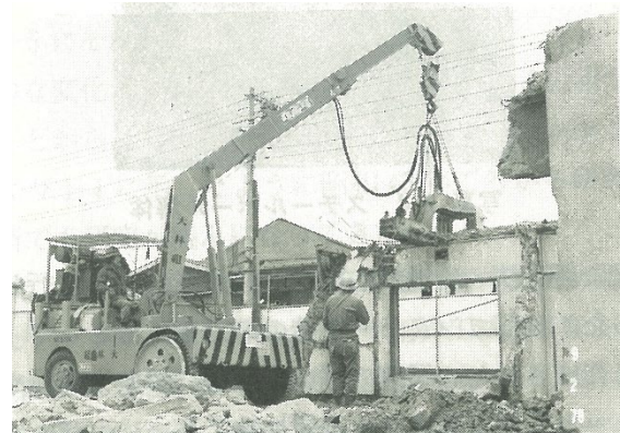
Photo 5 Crushing Method around 1978
