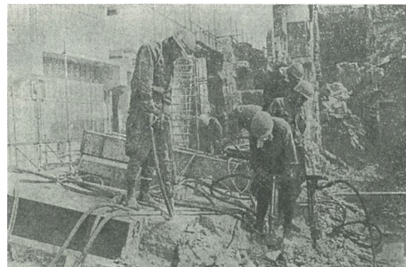
Photo 3 Demolitions due to a hand breaker (Bank of Japan Head Office around 1970)
