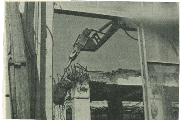
Photo 7 Demolition using a large breaker
